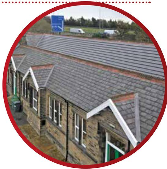
Our focus was on keeping as many of the original features as possible, which meant painstakingly removing all the original slate tiles so they could be reused on the new roof.
